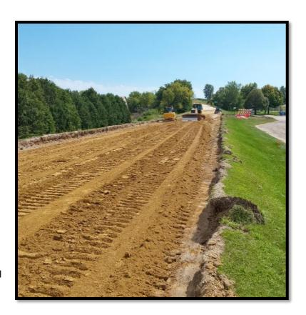
Thursday the grading crew completed geogrid and subbase placement on the rural portion of the project. In conjunction with that work, the crew tidied up the side street tie in areas in preparation for paving. Finally, the crew cored out  $4^{th}$  and  $5^{th}$  Ave. to the project limits.
