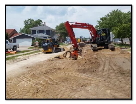
setting pipe to the north towards the existing manhole in the alley intersection just south of the gas station. The new pipe will be tied into this existing manhole and will be the northern endpoint of the sanitary sewer upgrades for this project.
